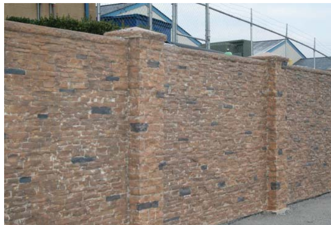
Above: One of Pour in Place's retaining walls.
