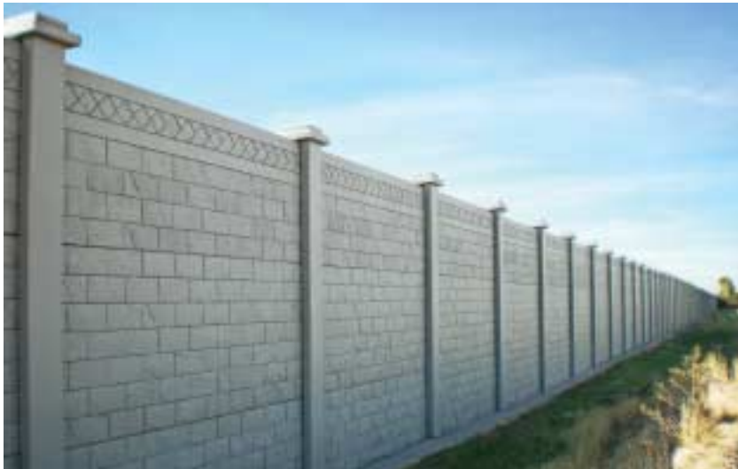
Fig. 2 The back side of the walls, which faces the residential area in its final position, features an ashlar slate design with a row of diamond shapes across the top section.
